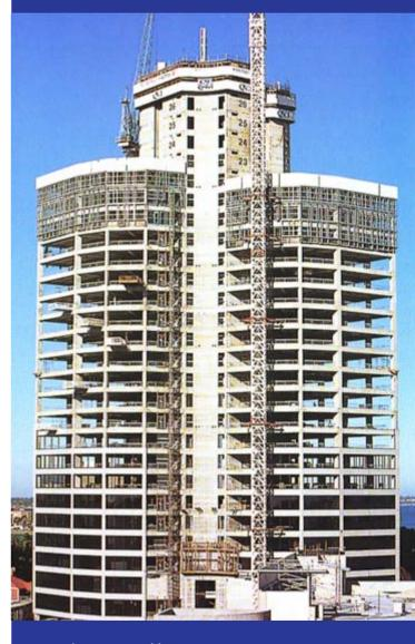
Typical Concrete Building Fame – economical, fast to construct and minimum storey heights.
