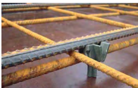
Figure 4. Mixing Class L mesh and Class N bars in a SSOW slab.
