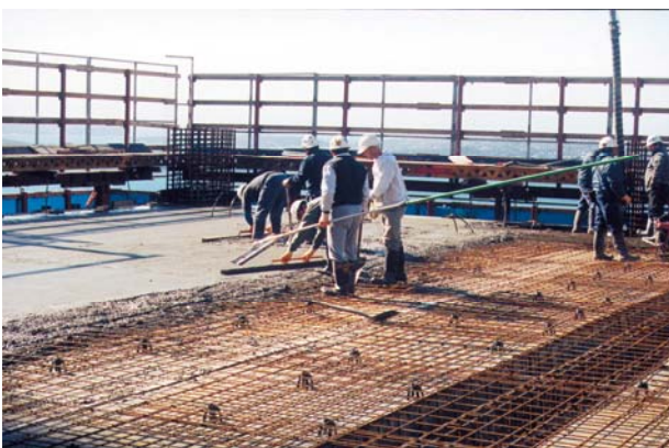
Figure 1 Examples showing low-ductility mesh being used in high-rise building construction
