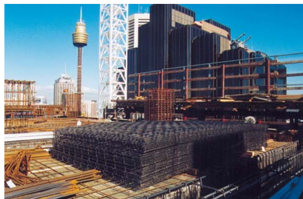
Figure 1 Examples showing low-ductility mesh being used in high-rise building construction
