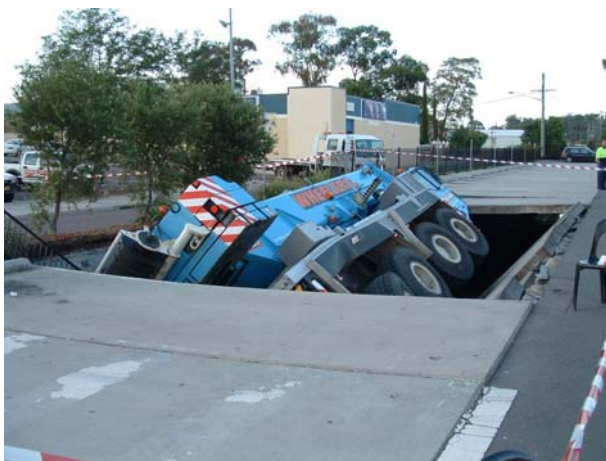
Figure 3 Sudden failure of severely overloaded slab, & deflection at failure in Australian tests
