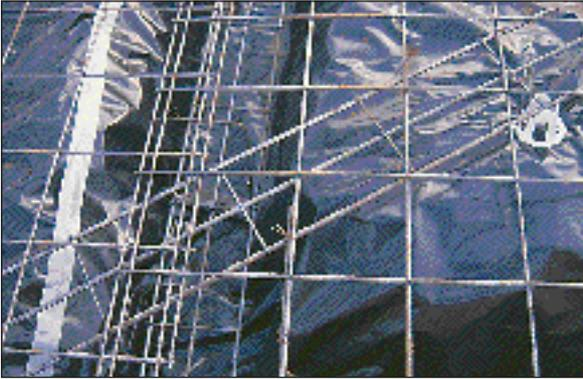
A slab-on-ground has thickened edges which are called edge-beams. Sometimes slabs also have internal beams which act as stiffening beams or wall supports. All these beams need steel reinforcement fixed near the bottom – this is called bottom-steel.
