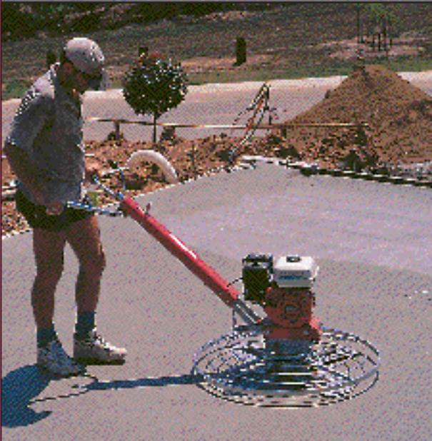
When the concrete compaction and screeding is done, the slab should be roughly floated with a trowel to give a smooth surface. After floating, the slab should be left to set hard enough so that a man standing on his heels will not sink more than 5 mm into the concrete.
