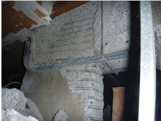
Figure 3: Failure of Beam/Column connection. Copthorne Hotel, Christchurch (Photograph courtesy Peter McBean, Wallbridge and Gilbert)
