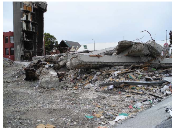
Figure 6: The shear wall remains standing amongst the ruins of the CTV Building, Christchurch, New Zealand (Photograph courtesy Peter McBean)
