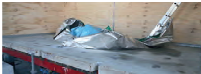
(a) Two-part proof-load test using water to 15 kPa (full height of tank), shown after test with liner wrapped up.
