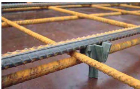
Figure 4. Mixing Class L mesh and Class N bars in a SSOW slab.
