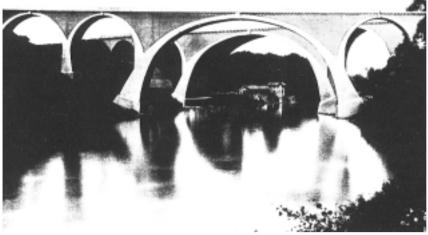
Figure 3 Plain concrete bridge at Kempten, West Germany, designed and built by Dyckerhoff and Widman in 1904; span 64.6 metres
