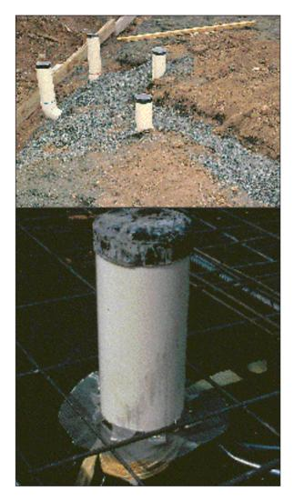
Drainage and water-supply pipes which are to be covered by the slab must be installed by a plumber at this stage.
