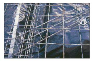
A slab-on-ground has thickened edges which are called edge-beams. Sometimes slabs also have internal beams which act as stiffening beams or wall supports. All these beams need steel reinforcement fixed near the bottom – this is called bottom-steel.
