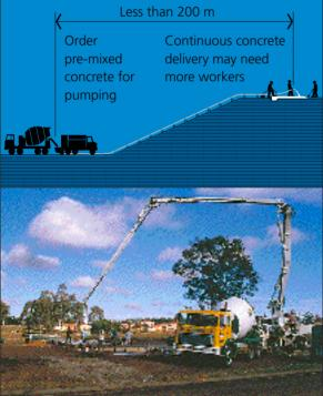
TOP Truck and pump for smaller slabs ABOVE Where longer reach is required use a truck-mounted pump with boom
