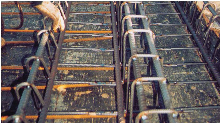
*The bond and anchorage properties of bars and mesh are not detrimentally affected by a light coating of rust which has formed on the steel surface after normal exposure to the atmosphere<sup>[1][2]</sup>.*
