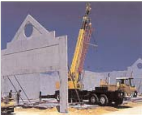
The speed of tilt-up construction is graphically demonstrated in these pictures of construction stages spanning only eight weeks
