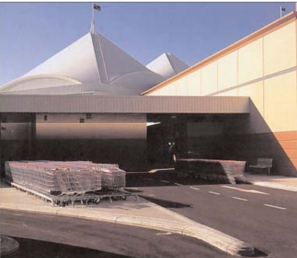
Tilt-up walls combine with the billowing roof of Lakeside Joondalup Shopping City
