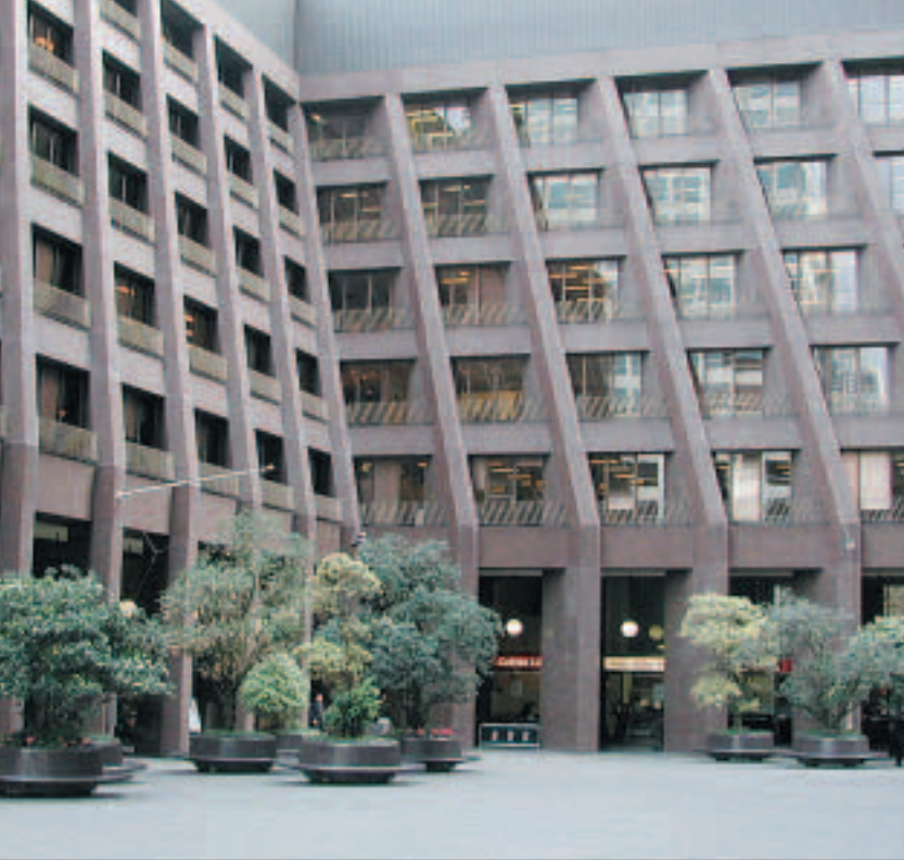
AMP Centre (Tower and St James Building), Melbourne – an example of a veneered facade from the 1960's
