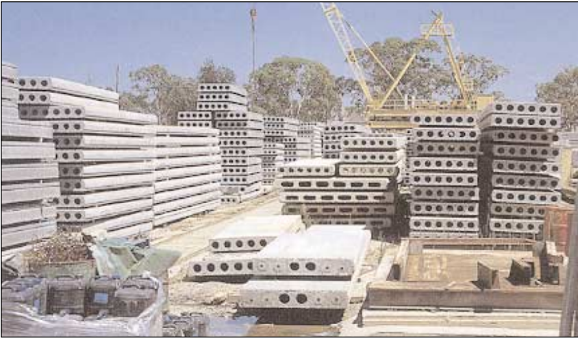
Panels, stored awaiting contractor's directions
