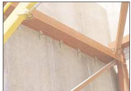
Typical top fixing, two cleats per panel
