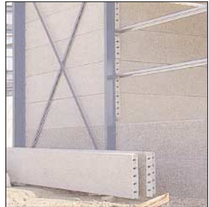
Technical and warehouse facility. Horizontal, exposed-aggregate-finish panels. Note use of dark river gravel in bottom panel to suggest plinth.
