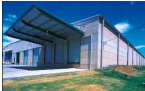
Over 2000 m 2 of fire-rated exposed aggregate hollowcore panels clad this warehouse for Southcorp at Arndell Park, NSW. A banding effect was achieved by using two colours of exposed aggregate.
