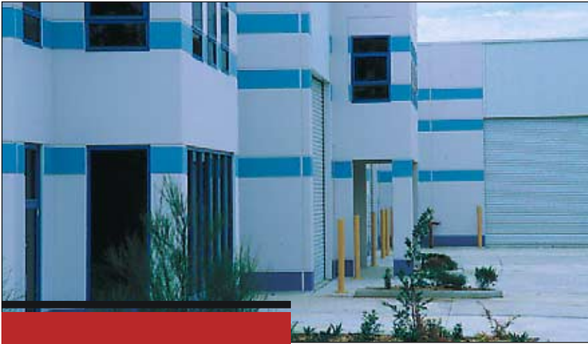
Factory-cast painted wall panels in industrial units, Lurnea, NSW
