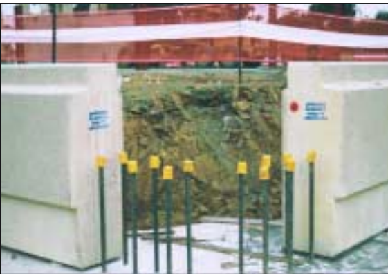
Starter bars for a loadbearing column connection
