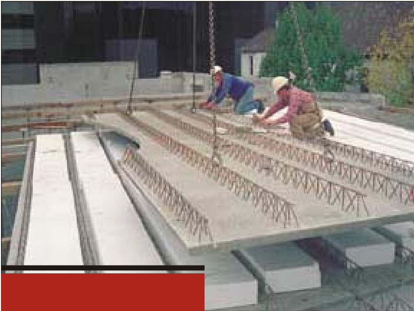
Semi-precast panels being placed on site
