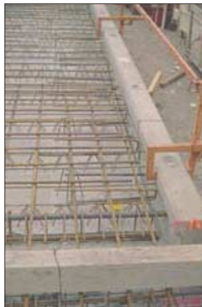
Transfloor panels connecting into a load bearing wall
