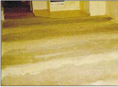
Thin coating of a proprietary self-levelling compound at panel joints where thin, flexible floor coverings are used
