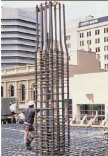
*Rivers Corporation Building, Adelaide, 1992. Prefabricated column cage incorporating seismic detailing. (Note close spacing of ties adjacent to floor and ceiling).*
