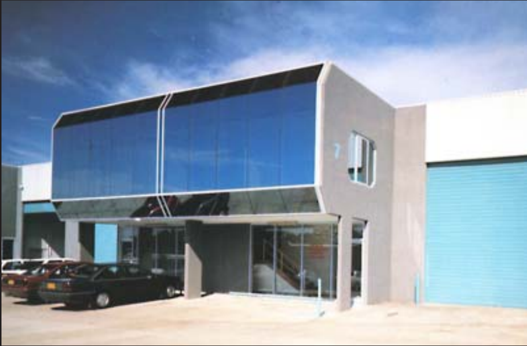
INDUSTRIAL ESTATE CASTLE HILL, NSW
