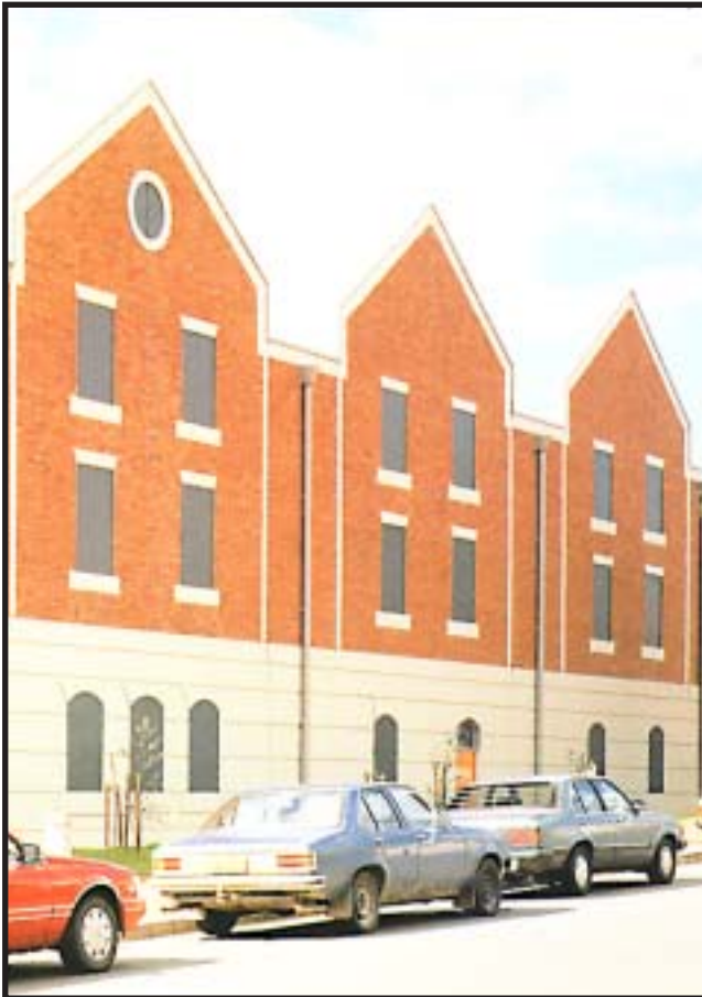
BRICK VANEER WALL PANELS
