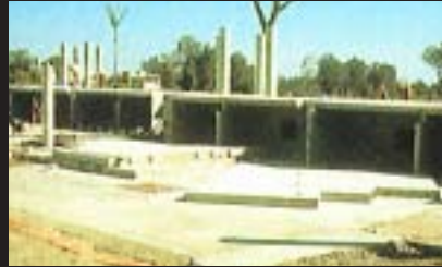
FIRST FLOOR PANELS POSITIONED
