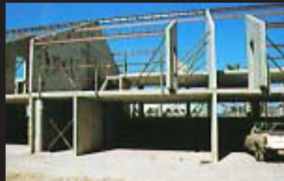
FIRST FLOOR WALL PANELS ERECTED
