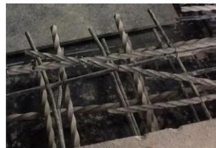
**Figure 8. Lapping of square twisted bars**
