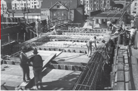
Construction of multi-storey flats in Sydney (ARC, 1953)
