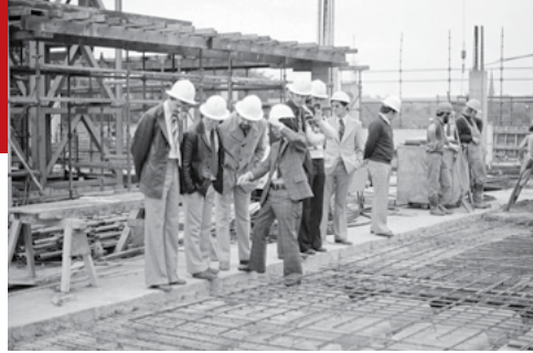
Inspection of reinforcement for Moonee Valley Grandstand (John Connell & Associates, 1977)
