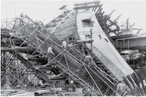
Sydney Opera House construction (Arup, April 1964)
