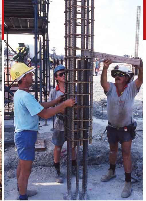
Installation of prefabricated cage in Robina, QLD (1994)
