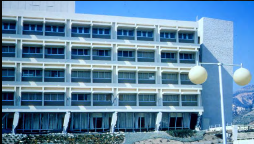
Failure of columns in San Fernando Earthquake, 1971 Olive View Hospital, California
