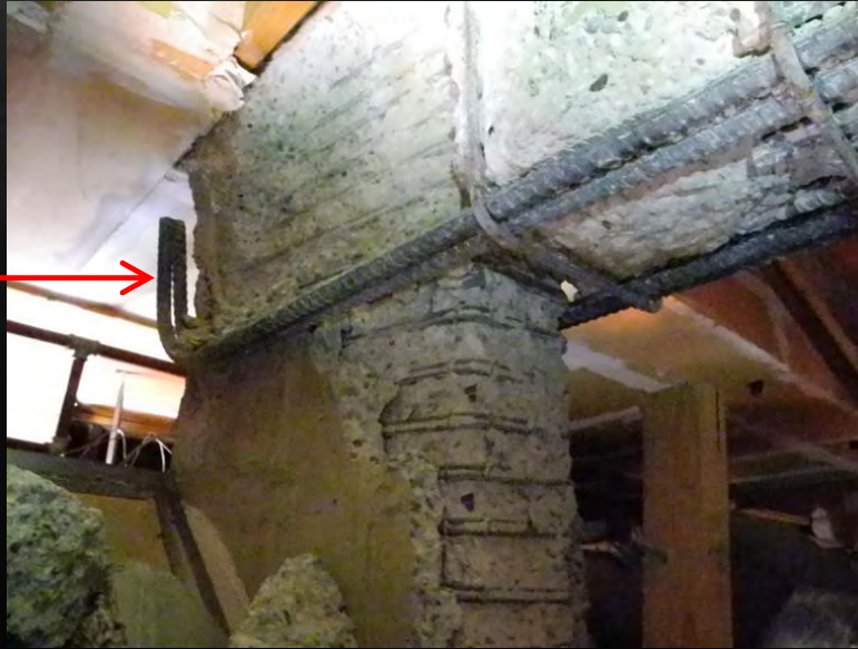
Failure of a transfer beam column joint at Cophthorne Hotel, Christchurch 2011
