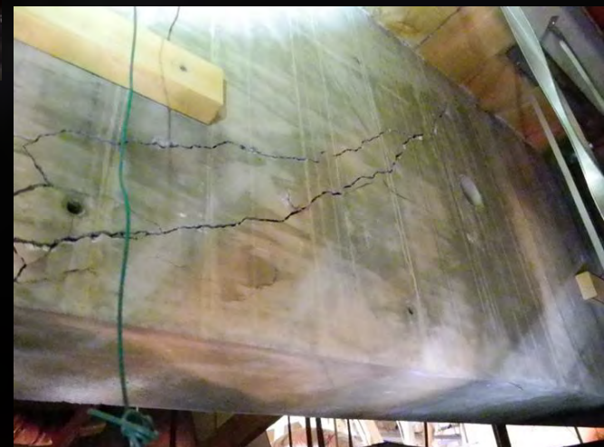
Failure of a transfer beam column joint at Cophthorne Hotel, Christchurch 2011
