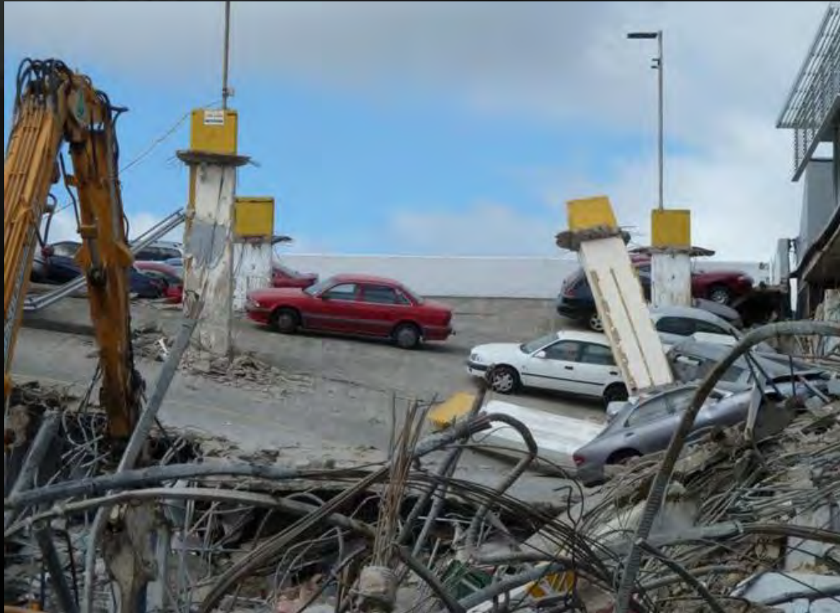
Remains of post-tensioned car park floor – Christchurch
